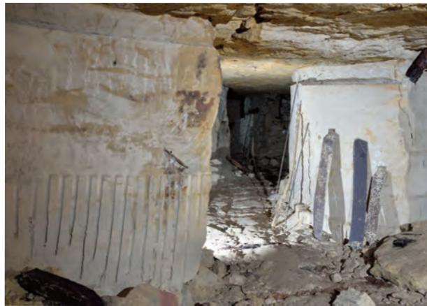
A view inside a bath stone mine, stacked up against the pillar are the original tools used. The wall on the left is studded with pick and tool marks.
